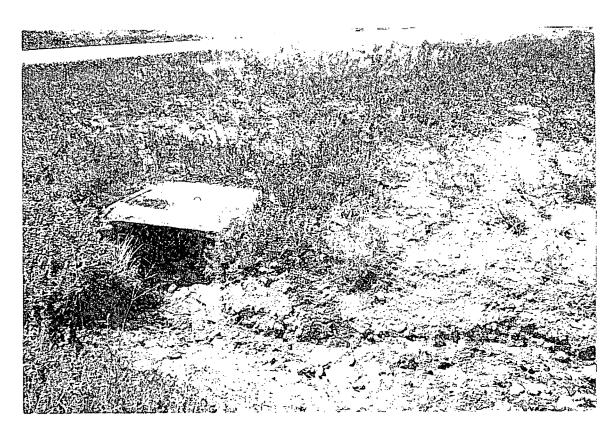
EXAMPLE OF SOIL EROSION DIRECTED TO STORMWATER PIPING
